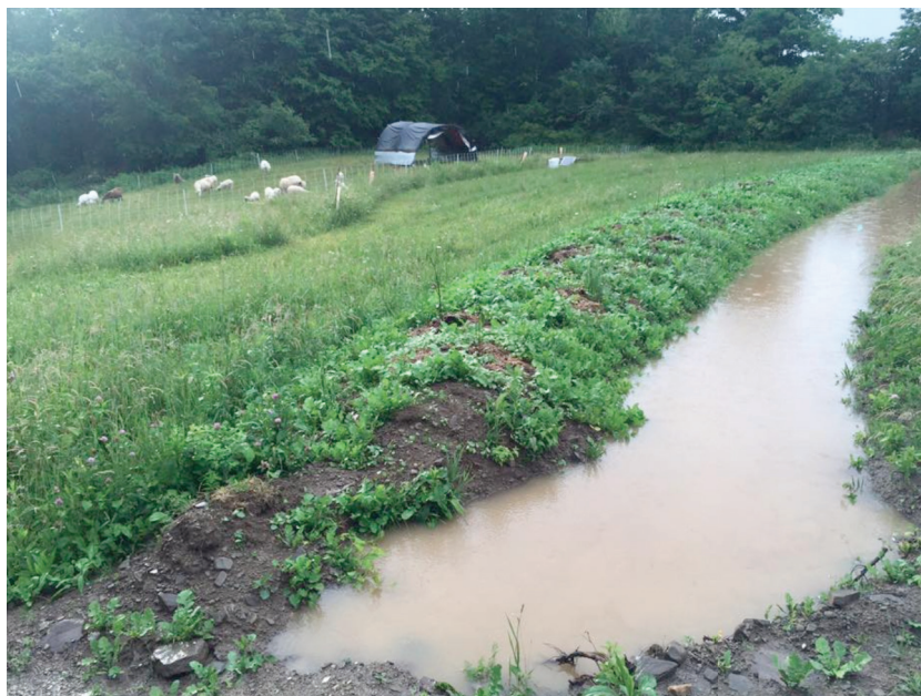
Full swale at Wellspring Forest Farm, soon after installation.
